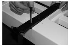
Attach the strap with the pins to the front side of the gate using carriage bolts. Pass the bolts through the strap, both back plates, and secure with washers and nuts. Secure firmly but do not over tighten. Depending on the thickness of the gate, the bolts may have to be trimmed. The slot in the strap hinge allows for lateral adjustment (ideally the blot should be in the center of the slot which allows for a full half inch of lateral movement in each direction).
