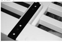
Place the first strap back plate so the bend hooks around the edge of the gate upright (stile) on the hinge side. It should be centered on the horizontal rail. Attached the back plate to the gate using two screws. If the rails are a different thickness to the stiles then it will be necessary to use filler blocks. We suggest a solid cellular pvc product such as azek.
