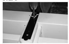
Flip the gate over and attach the second back plate on the other side so it is at the same level (measure down from the top of the gate so that the distance is the same on both sides) as the first back plate. Drill holes and fasten as in Step 2 above.
